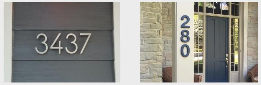
House address numbers shall be 4" minimum high,  $\frac{1}{2}$ " stroke width visible from the street. Missing numbers shall be replaced. May be located on either house or mailbox.
