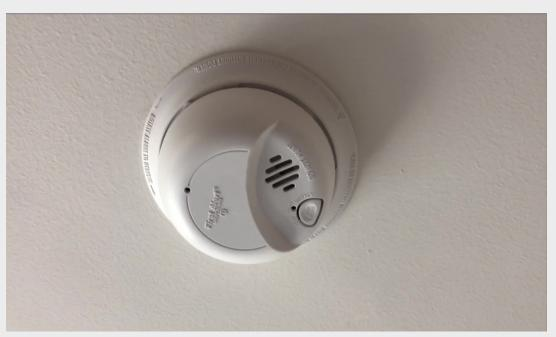
Smoke detectors must be installed in each bedroom, in each hall in the immediate vicinity of bedrooms, and on each floor level of the structure. (main floor, any usable attic or 2nd floor space, any usable basement; not an in-accessible attic). Smoke detectors may be battery operated, but existing hard-wired systems must be maintained.
