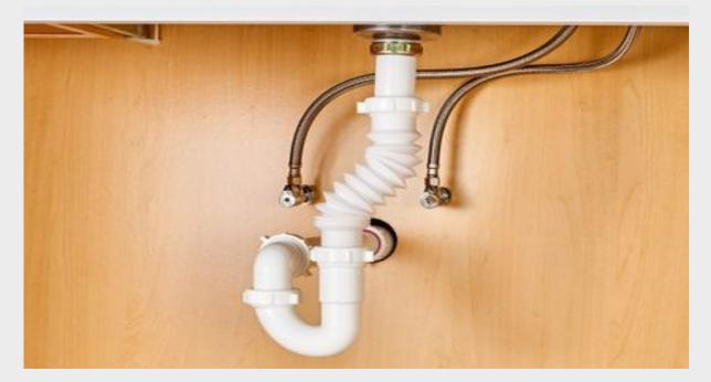
Flex piping on drains is not allowable, per Plumbing requirements. Unvented sinks and vanities will be required to be properly vented by a licensed plumber.
