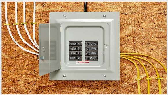
Minimum 60 amp service is allowable. Inspectors check cable clamps and circuits for appropriately rated fuses. Inspector opens box door, but does not remove the box cover to verify circuit installations inside the box.
