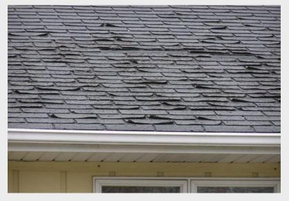
Deteriorated overhang, loose or missing roof shingles, roof flashing and vents shall be repaired/replaced. Roofs leaking badly will require a full replacement.
