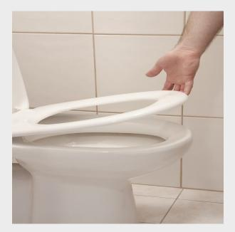
Check toilet anchorage to the floor. Check for a secure toilet seat. Defective toilet flush mechanisms shall be repaired/replaced to ensure proper water level. Check seal at toilet base for leakage.
