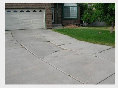
Surface differentials of <sup>3</sup>/<sub>4</sub>" or more on driveways and walkways are a trip hazard and must be leveled. <sup>3</sup>/<sub>4</sub>" cracks must be repaired. Gravel driveways must come into compliance with city code.
