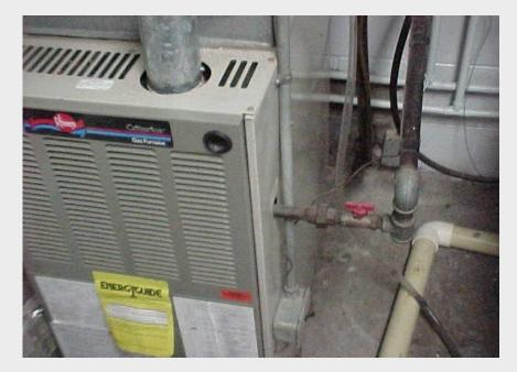
Check for natural gas shut-off valves on the furnace, water heater, stove/oven and ranges. Each appliance must have a separate shut off valve within 6 feet of appliance.
