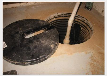
Cannot drain into existing sanitary sewer; must drain to the exterior. Drainage/ Underground drainage must be keep back 15' from the backside of street curb. No extension cords; not installed per manufacturer's instructions. No GFCI required.
