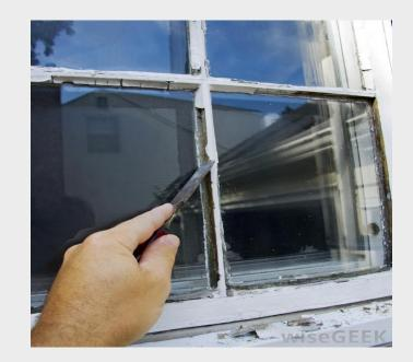
Window sash must operate freely and stay open when lifted. Glazing must be maintained free from cracks and voids.
