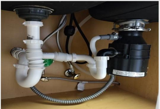
Flex piping on drains is not allowable, per Plumbing requirements. Unvented sinks and vanities will be required to be properly vented by a licensed plumber.
