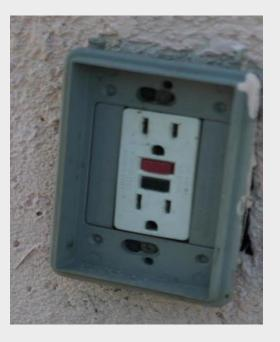
Exterior outlet receptacles shall have waterproof covers and be protected on a ground fault circuit interrupter (GFCI) circuit. (The photo on the right would be unacceptable.) We do require GFCI outlets in an existing garage
