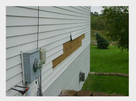
Check for melted, deformed, damaged and missing siding.
