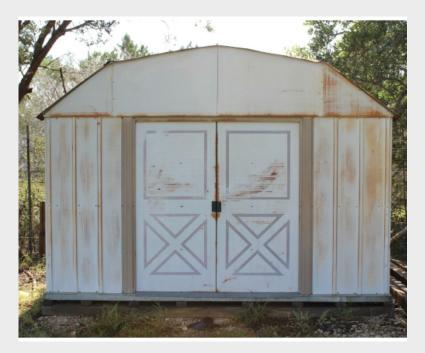
All exterior surfaces where chipping and peeling paint occurs shall be scraped and painted. Accessory structures shall be maintained structurally sound and in good repair.
