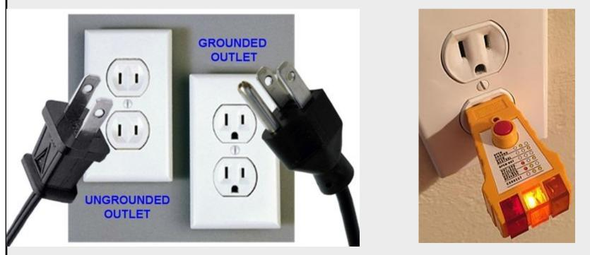
Inspectors check for open grounds and improper wiring with a tester on receptacle outlets. Original two-prong systems are acceptable, if maintained. Three-prong outlets not grounded must be properly grounded, or switched back to two-prong.
