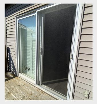
Every window, sliding door, and other outside opening required for ventilation of habitable rooms shall have tightly fitting screens.
