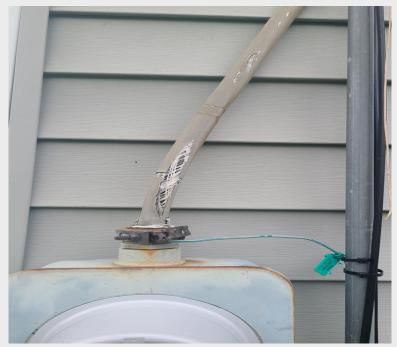
Any deteriorated and defective entry cable must be replaced under permit to eliminate hazards. If outer sheathing of cable is frayed or deteriorated, we cite.
