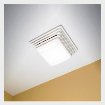
Bathrooms must have an operable window, or a mechanical exhaust fan. Exhaust fans must vent to the exterior and be located at the top of a wall or in the ceiling.
