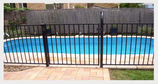
Pools, hot tubs and spas must be surrounded by a 4 foot high fence or barrier and use gate latch hardware not accessible to small children. Gates are required to be self-closing and self-latching from a still position 6" from the gatepost. Where self- latching device is less than 54 inches above the bottom of the gate, the release mechanism shall be located on the pool side of the gate.
