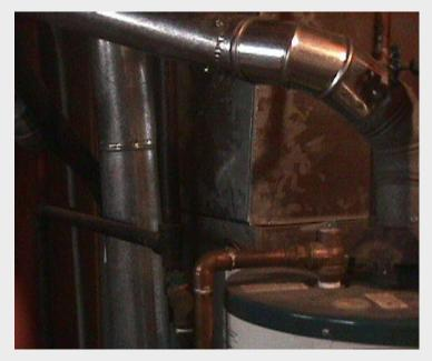
No bright (flimsy) aluminum vent; must be dull (sturdy) galvanized venting.
