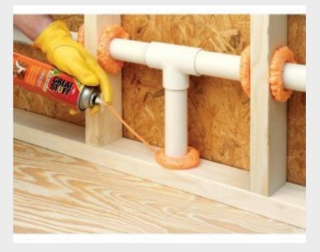
No spray foam products are allowable. Fire-rated caulk may be acceptable, if applied in a workmanlike manner.
